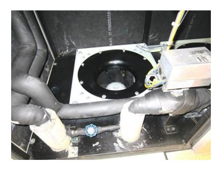
Note: Impeller under the floor for better air flow
