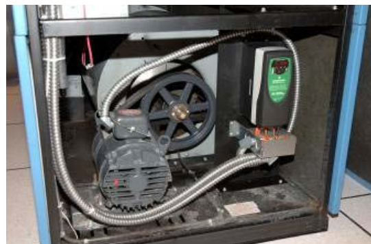
Figure 5: VFD installed.
