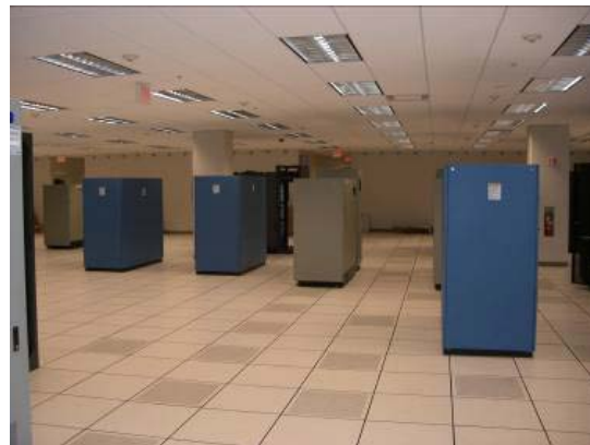
Figure 4: Open floor tiles.
