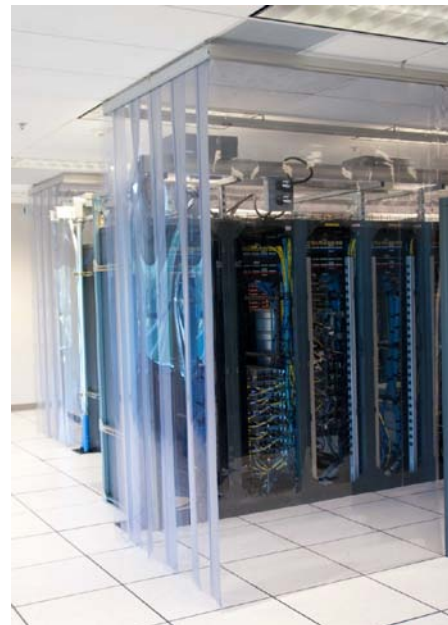
Figure 7: hot-aisle containment curtains.
